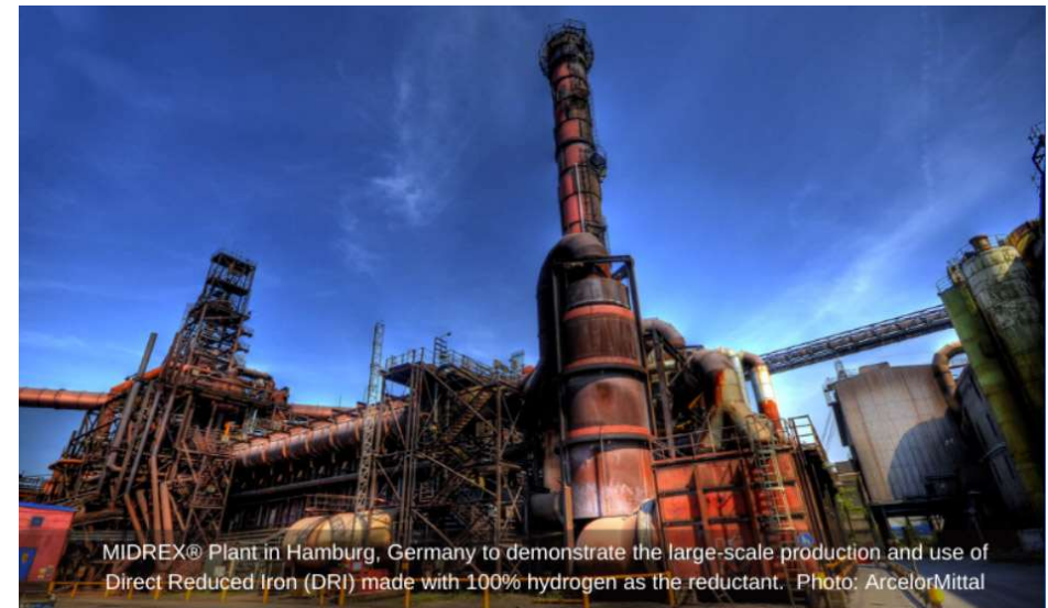
Demonstration plant for H 2 -based DRI
