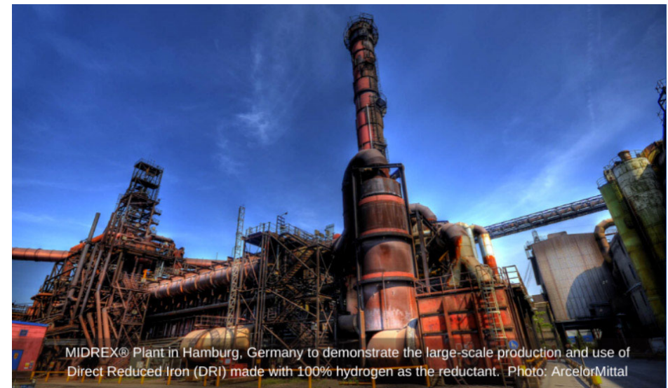
Demonstration plant for H 2 -based DRI
