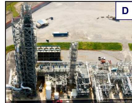
500TPD大型実証機(Southern Company)
