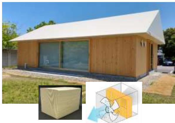
DAC実験棟 (RITE敷地内設置)
