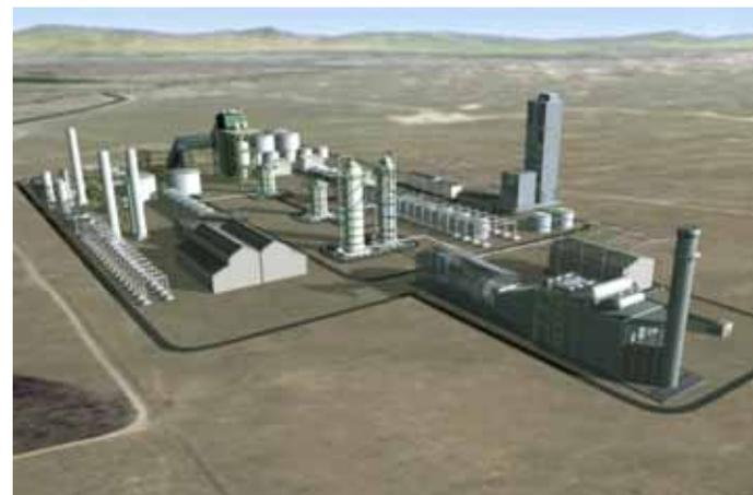
IGCC with Hydrogen Turbine and Full Integrated Carbon Capture & Sequestration
