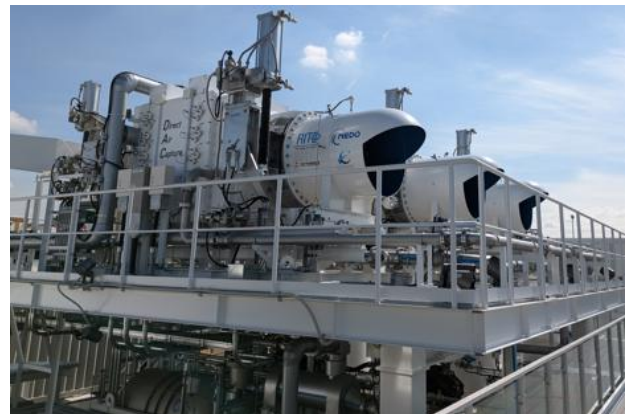
Fig. 3. Pilot-scale demonstration test equipment installed at the Osaka-Kansai Expo site
