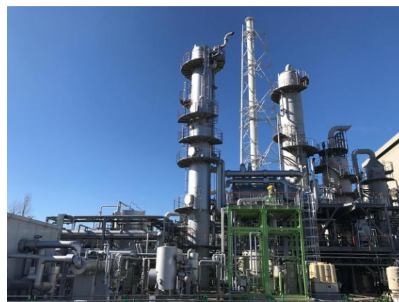
Fig. 10. Equipment of energy-saving CO 2 absorption process ESCAP® at Niihama Nishi Power Station, Sumitomo Joint Electric Power Co., Ltd.
