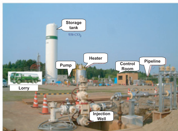
Iwanohara demonstration test site
