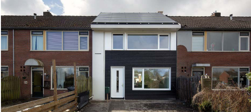
Netherlands: Energiesprong prefabricated thermal retrofits, net-zero housing
