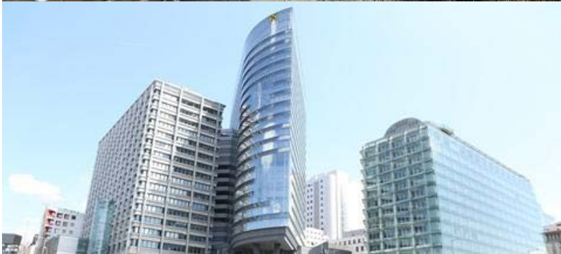
Austria: Raiffeisen First Passivhausstandard office tower retrofit
