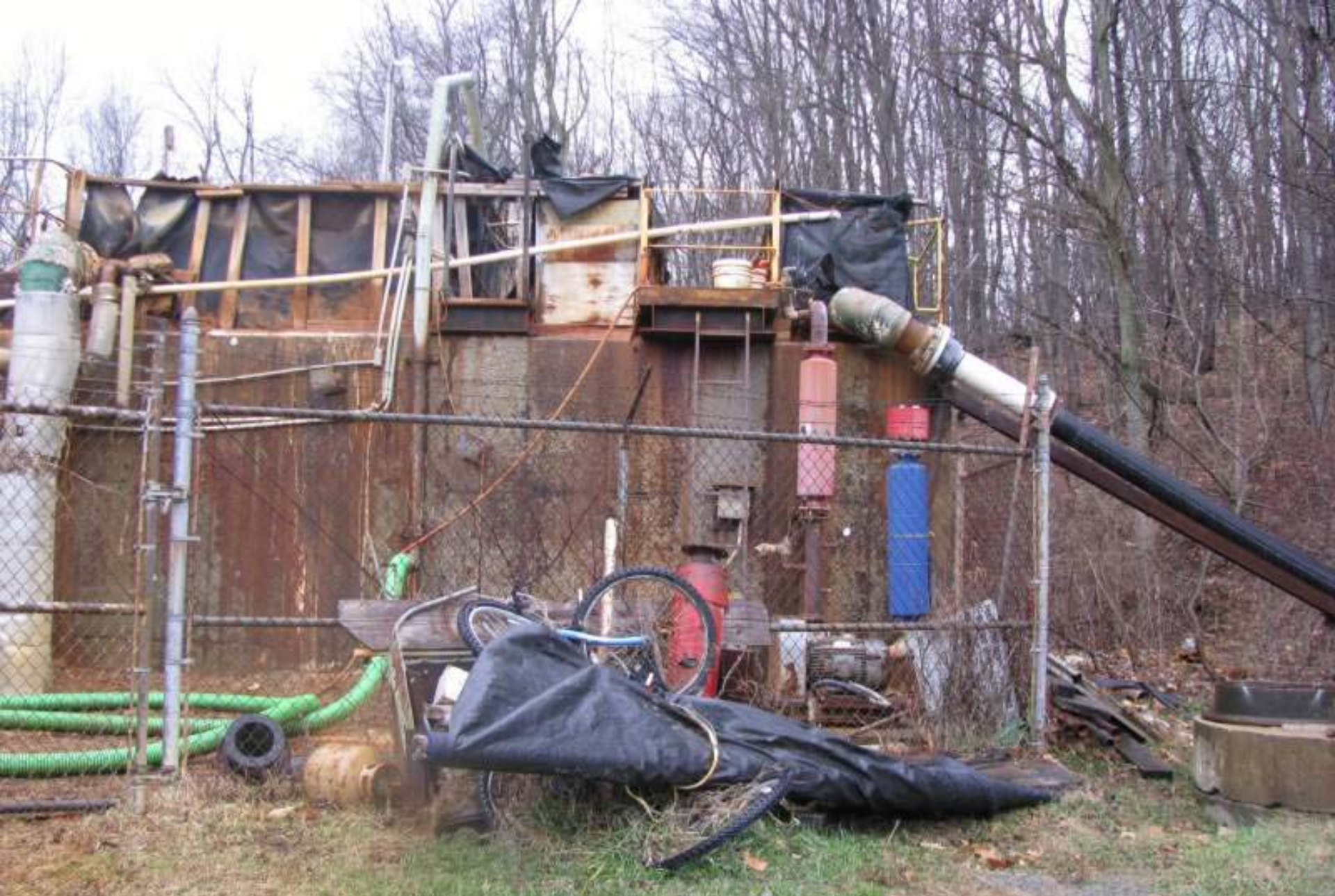
Brine Treatment Plant – Conemaugh River
