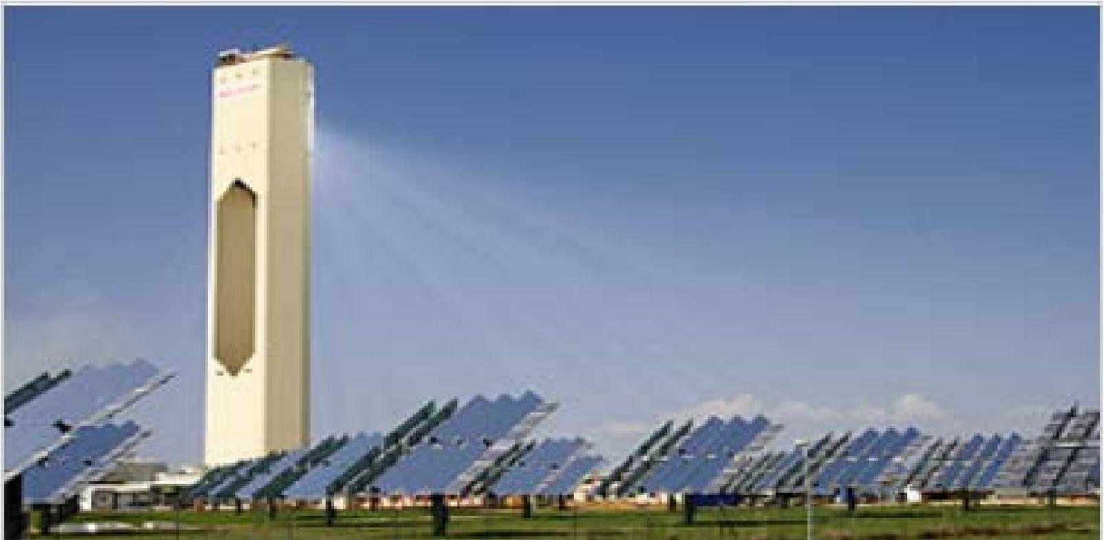
The **PS10 solar power plant** in Andalucía, Spain, concentrates sunlight from a field of **heliostats** onto a central **solar power tower**.
