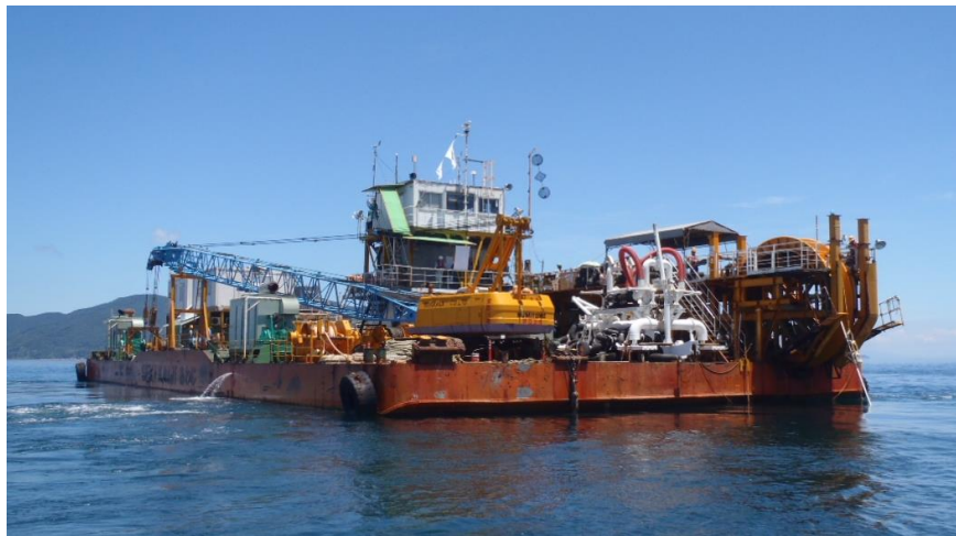
Salvage barge for cable burial
