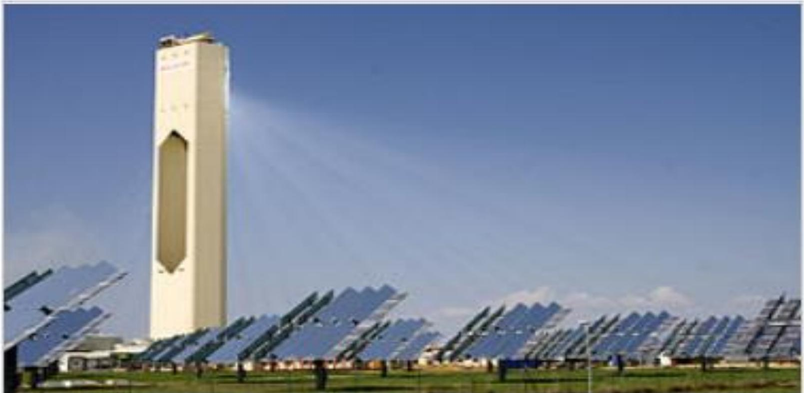
The **PS10 solar power plant** in Andalucía, Spain, concentrates sunlight from a field of **heliostats** onto a central **solar power tower**.
