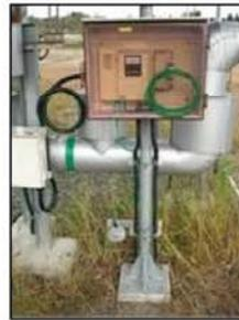
CO<sub>2</sub> detector (No leak)
