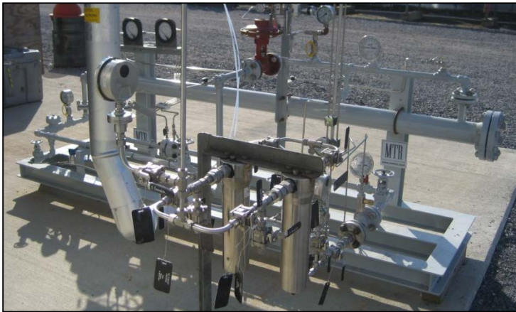
Bench-scale module test skid
