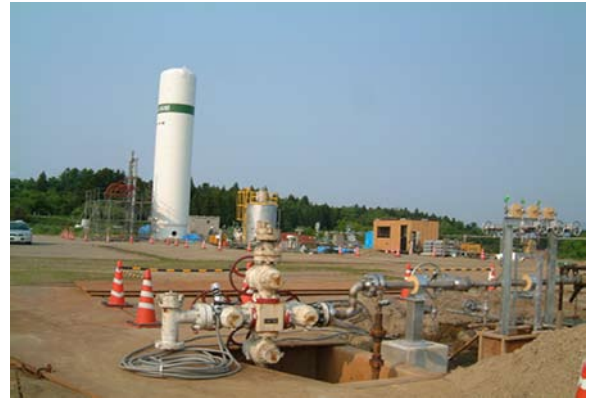
Fig2 CO 2 injection facilities at Nagaoka site
