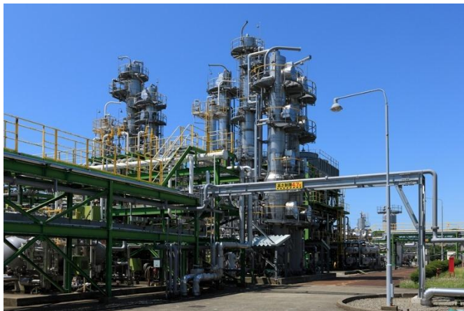
Natural Gas Plant
