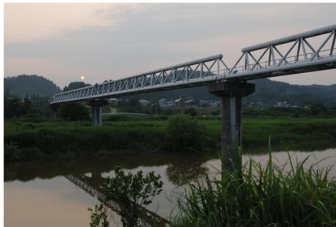
Gas Trunk Line over a river
