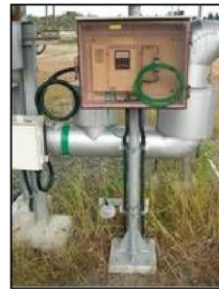
CO 2 detector (No leak)
