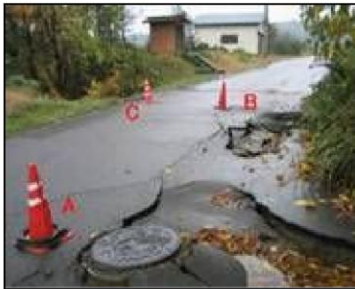
Access road was damaged.
