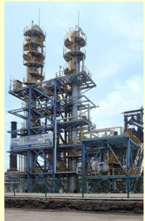
Chemical absorption pilot Plant (COURSE50: NEDO Project) Source: Nippon Steel Eng. HP.
