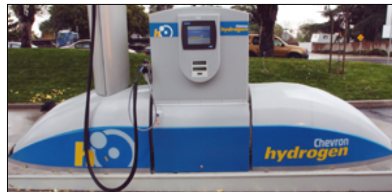
Hydrogen Fueling Dispenser
