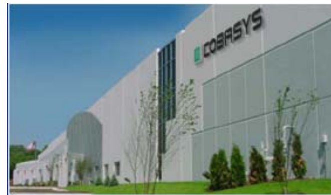
New Manufacturing Facility Springboro, Ohio
