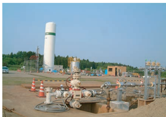
Fig.2 CO 2 injection facilities at Nagaoka site
